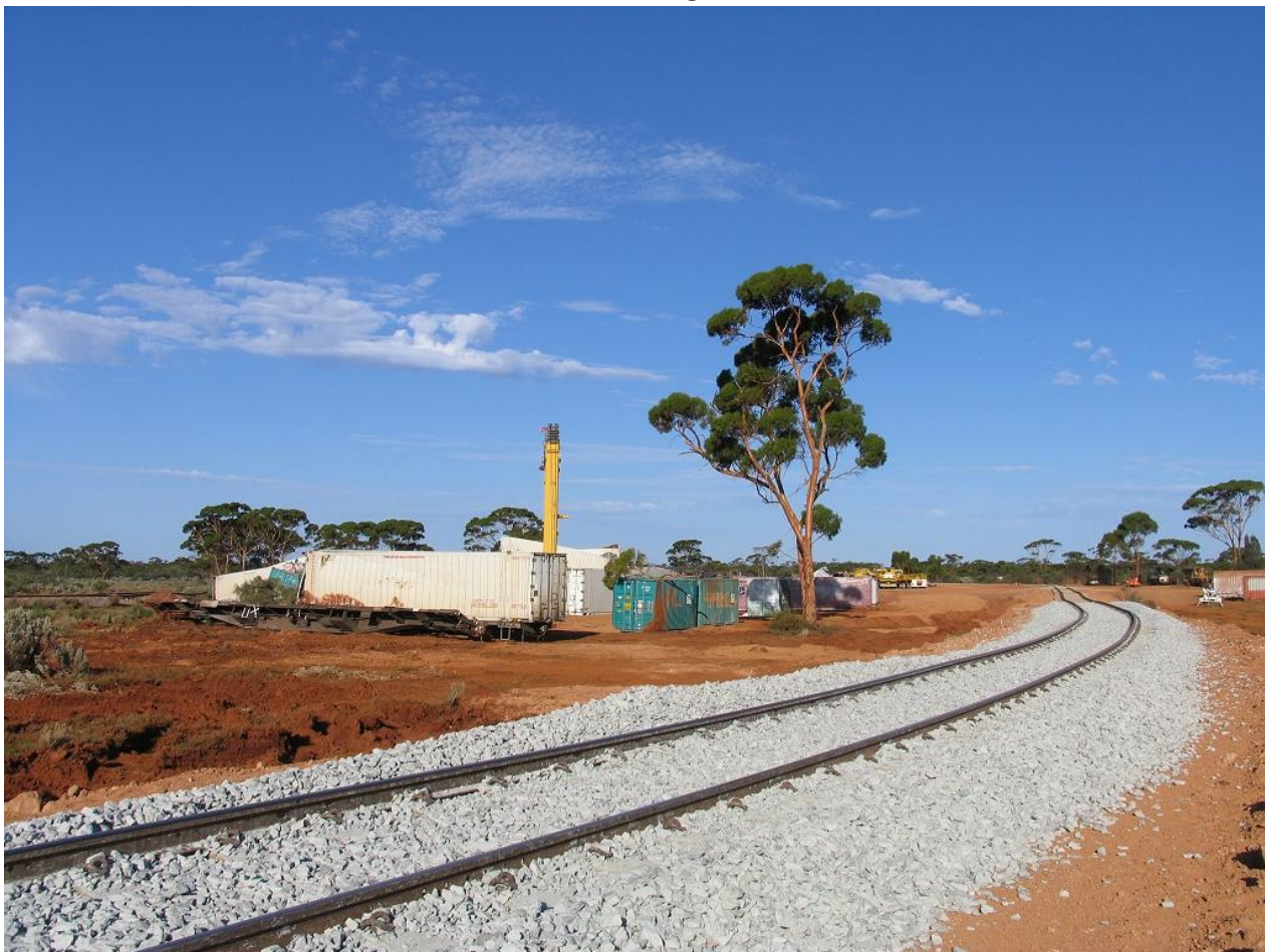
Partially ballasted deviation with recovery of 5PS6 loading underway on 5th. Photo John Bollans
