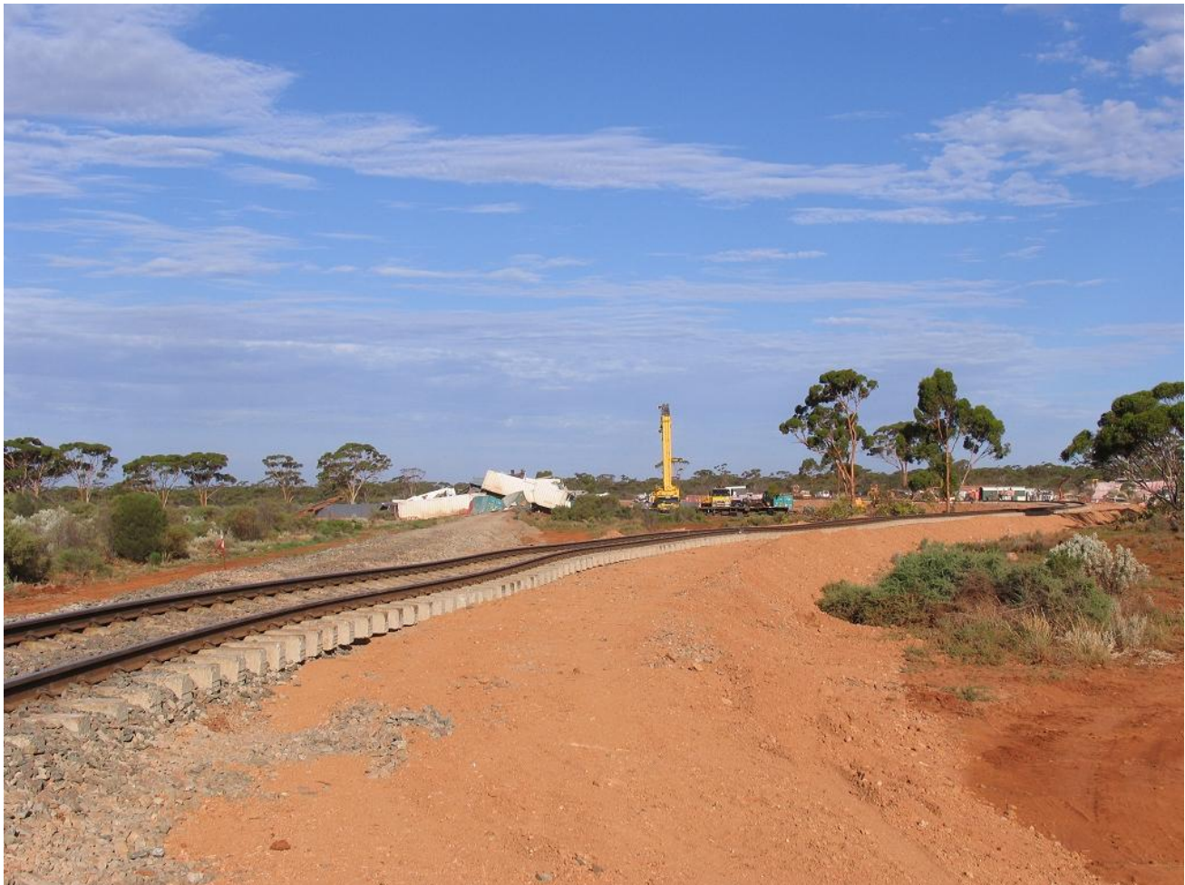
Completed deviation and slewed main line track at 5PS6 derailment on 4th February. Photo John Bollans
