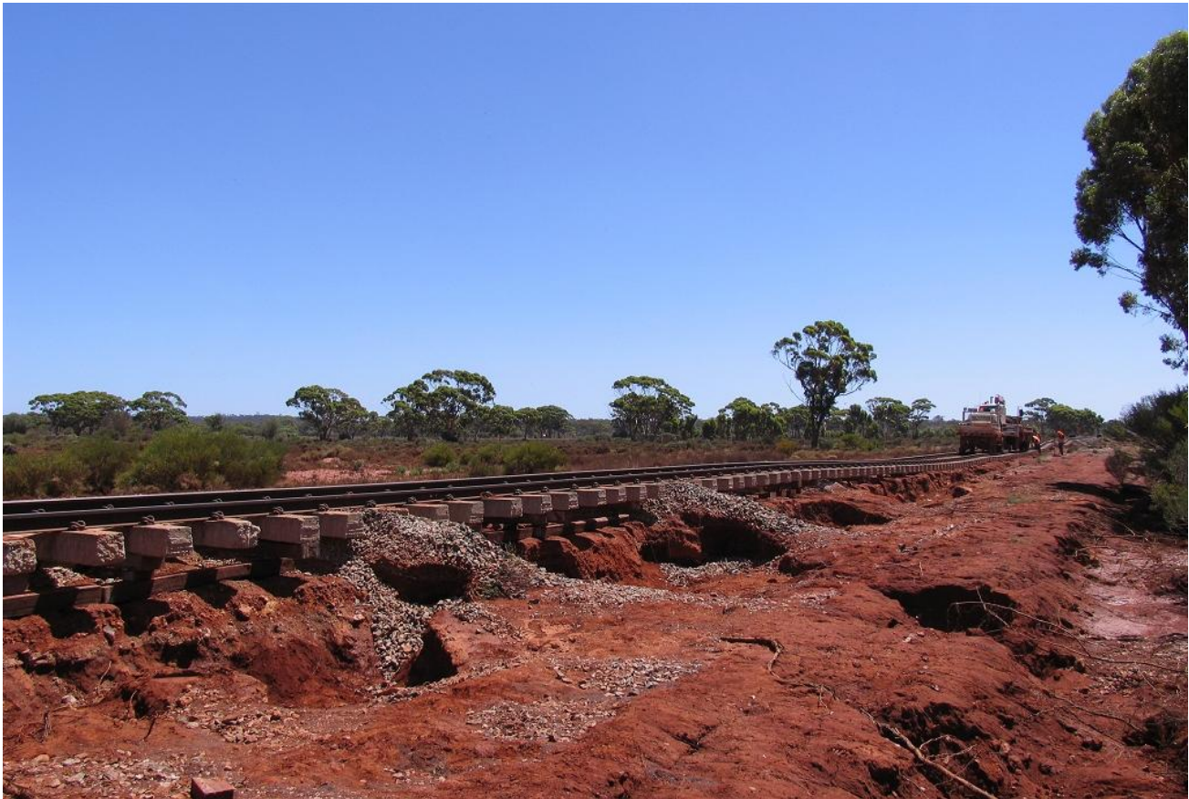
Washaways with the deep scouring of the embankment and track bed are east of the 1738.600km derailment site with these washaways under repair on 1st February. Photo John Bollans
