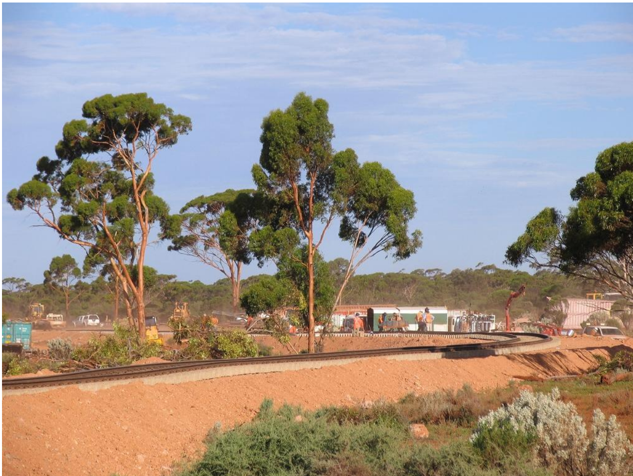
Unballasted deviation at 1738.600km where ballasting commenced at 2100 on 4th. Photo John Bollans.
