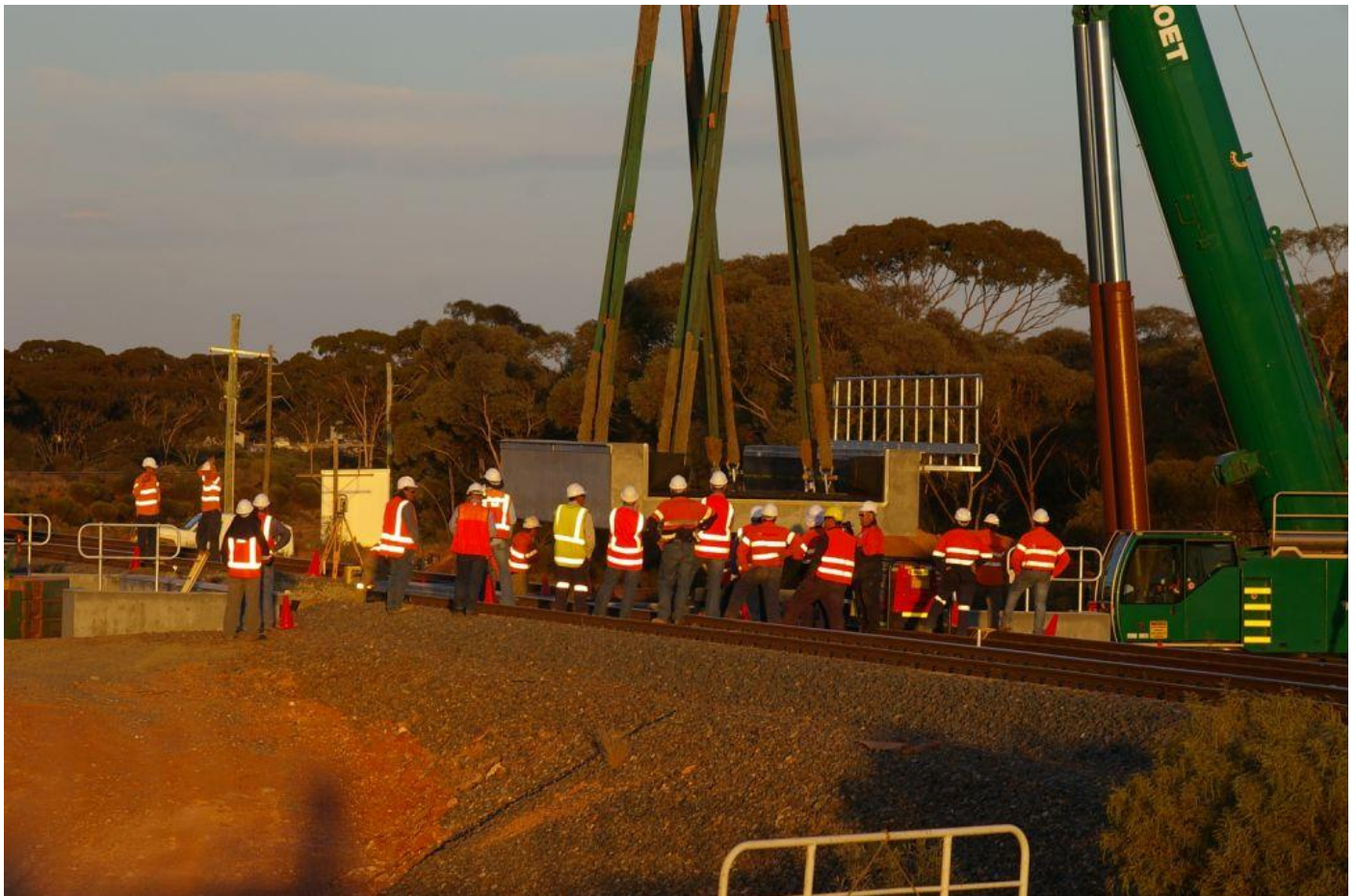
Esperance line span is lowered into place just on dusk with the new bridge over a mine haul road put in place in less than 12 hours giving minimal disruption on these important heavy traffic lines. Photo Peter Donaghy
