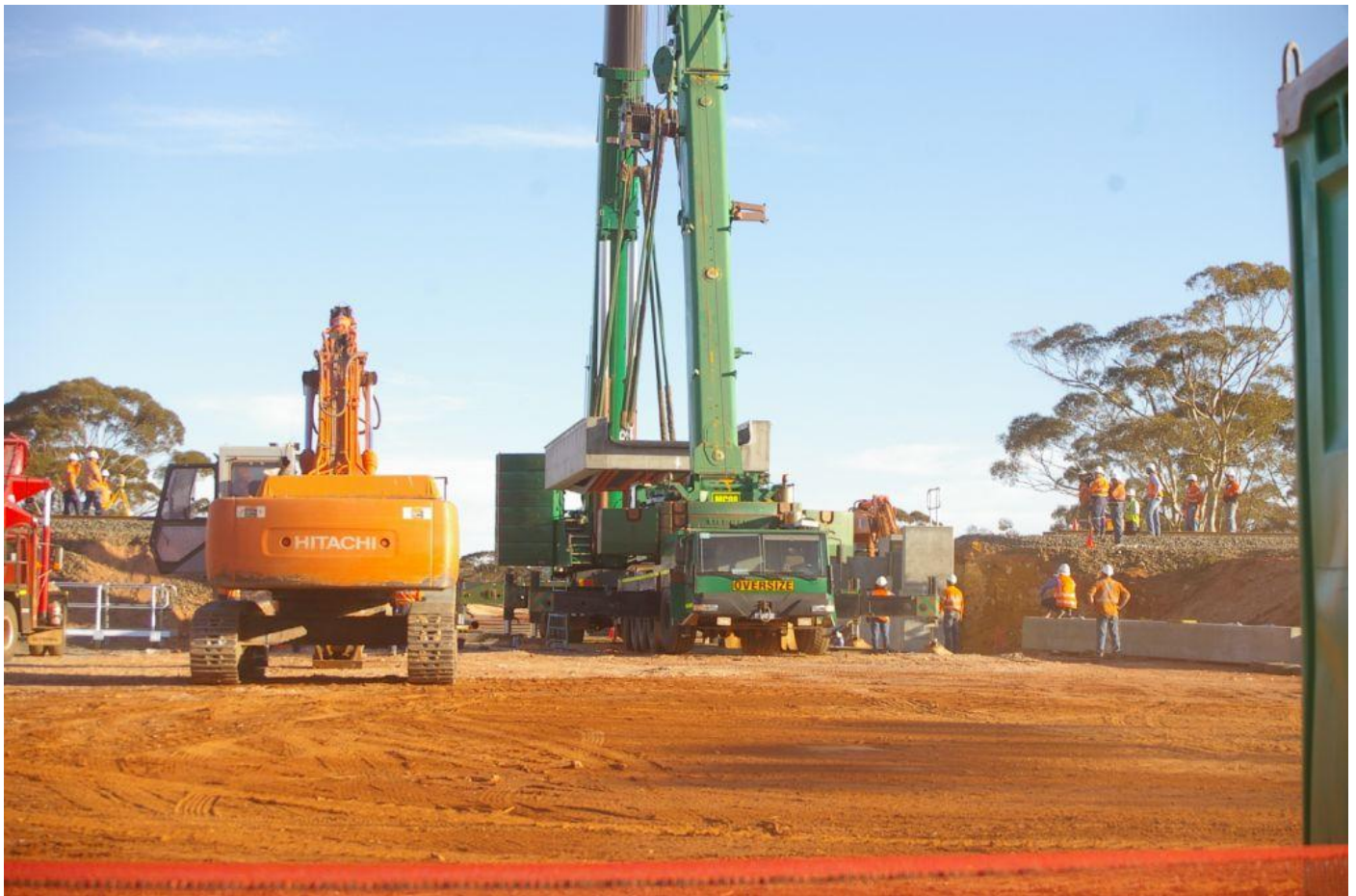
200 tonne and 500 tonne crane prepare to lift main span on to EGR line at Binduli on November 3rd.
