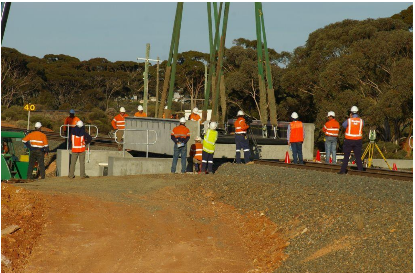
EGR main line span is being lowered into place in the late afternoon of the 3rd. Both photos Peter Donaghy
