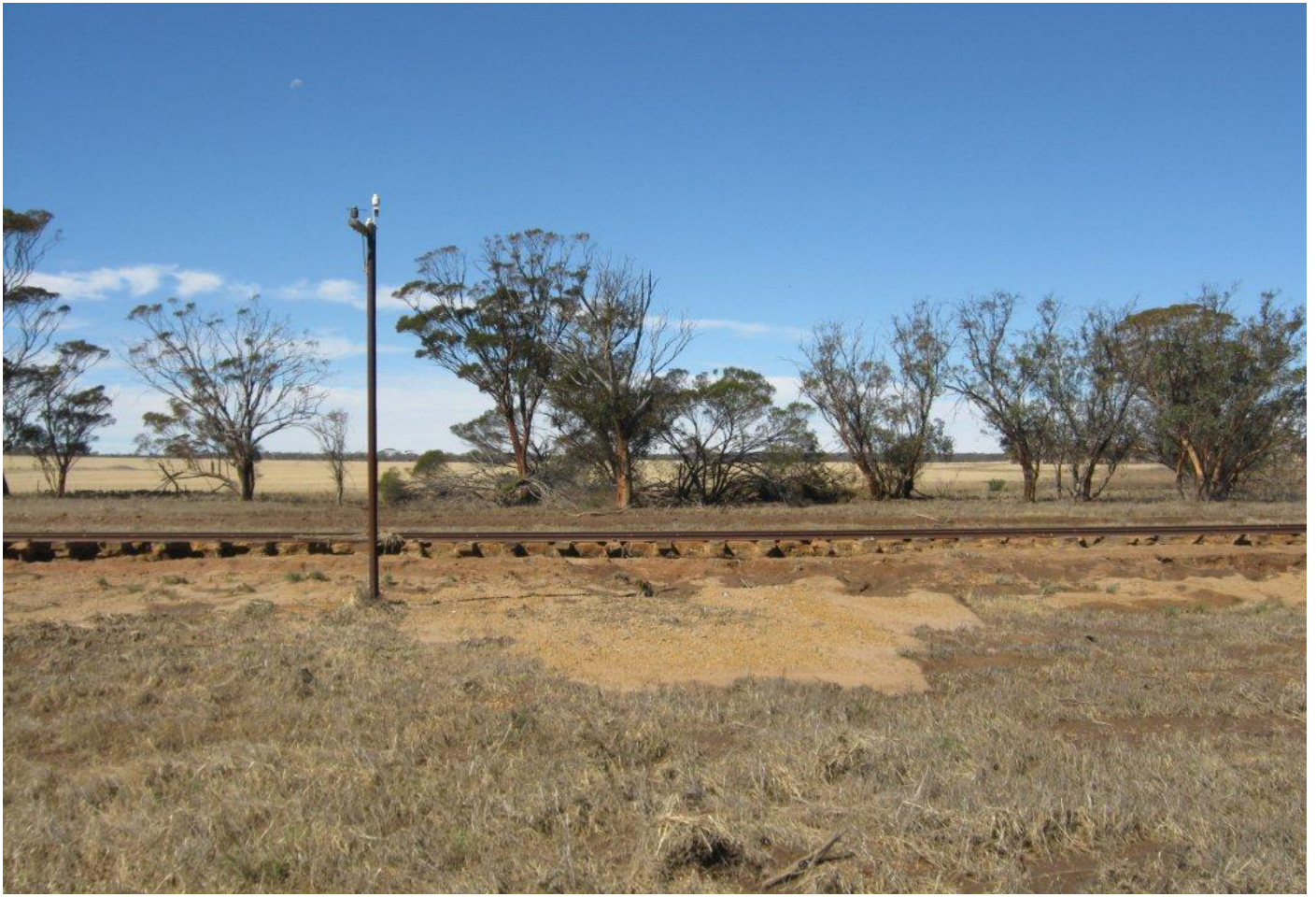
Damage on February 12th Merredin to Nungarin line that was caused by the flash flood. Photo Justin Smith
