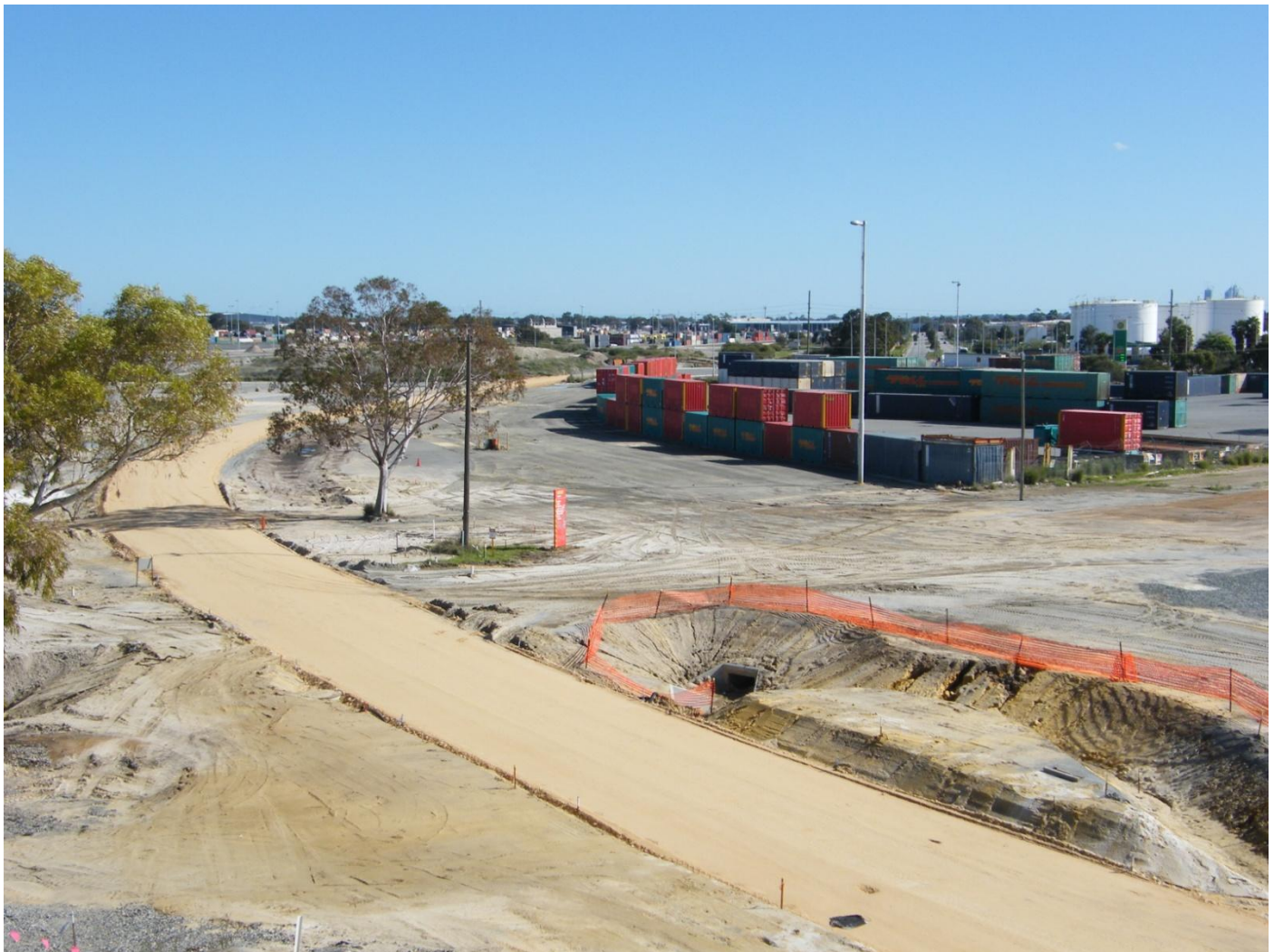
Formation for new access to BP terminal and PTA Kewdale bypassing diagonal July 17th. Photo Jim Bisdee
