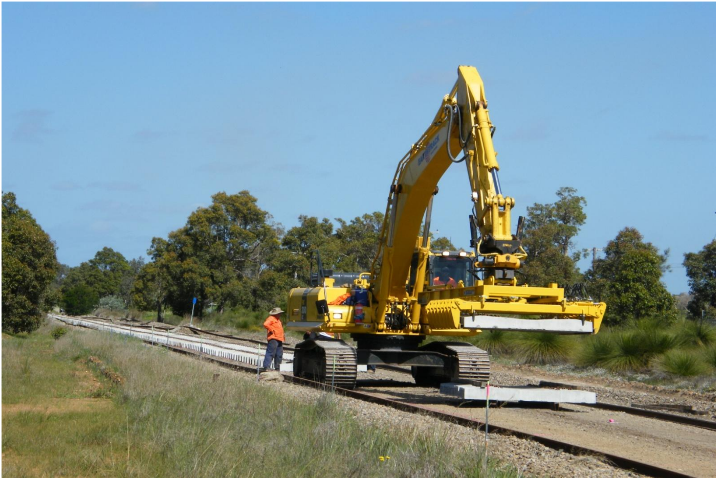
Sleeper placing machine picking eight sleepers to be placed on track bed at Byford on September 8th.
