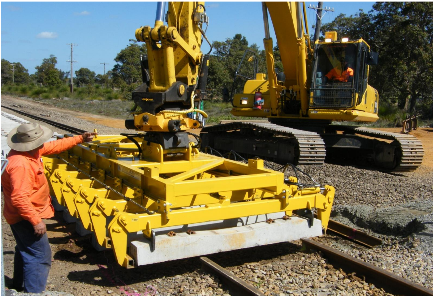
Sleepers being placed on the track bed at Byford on September 8th.
