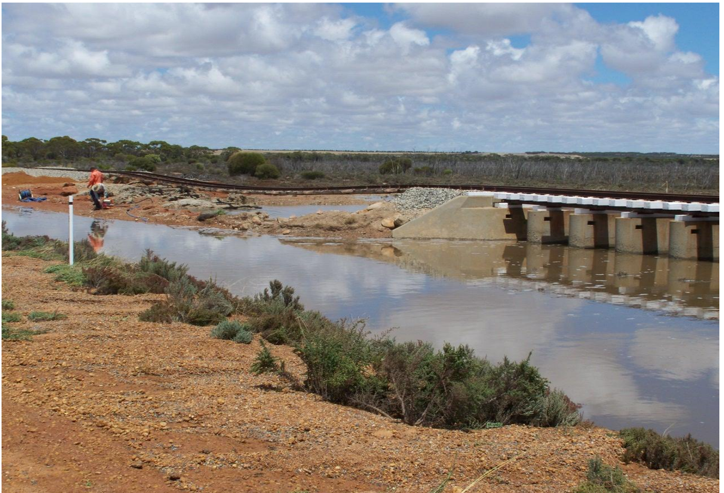
Track washed away at Pingaring floodway December 10th.
