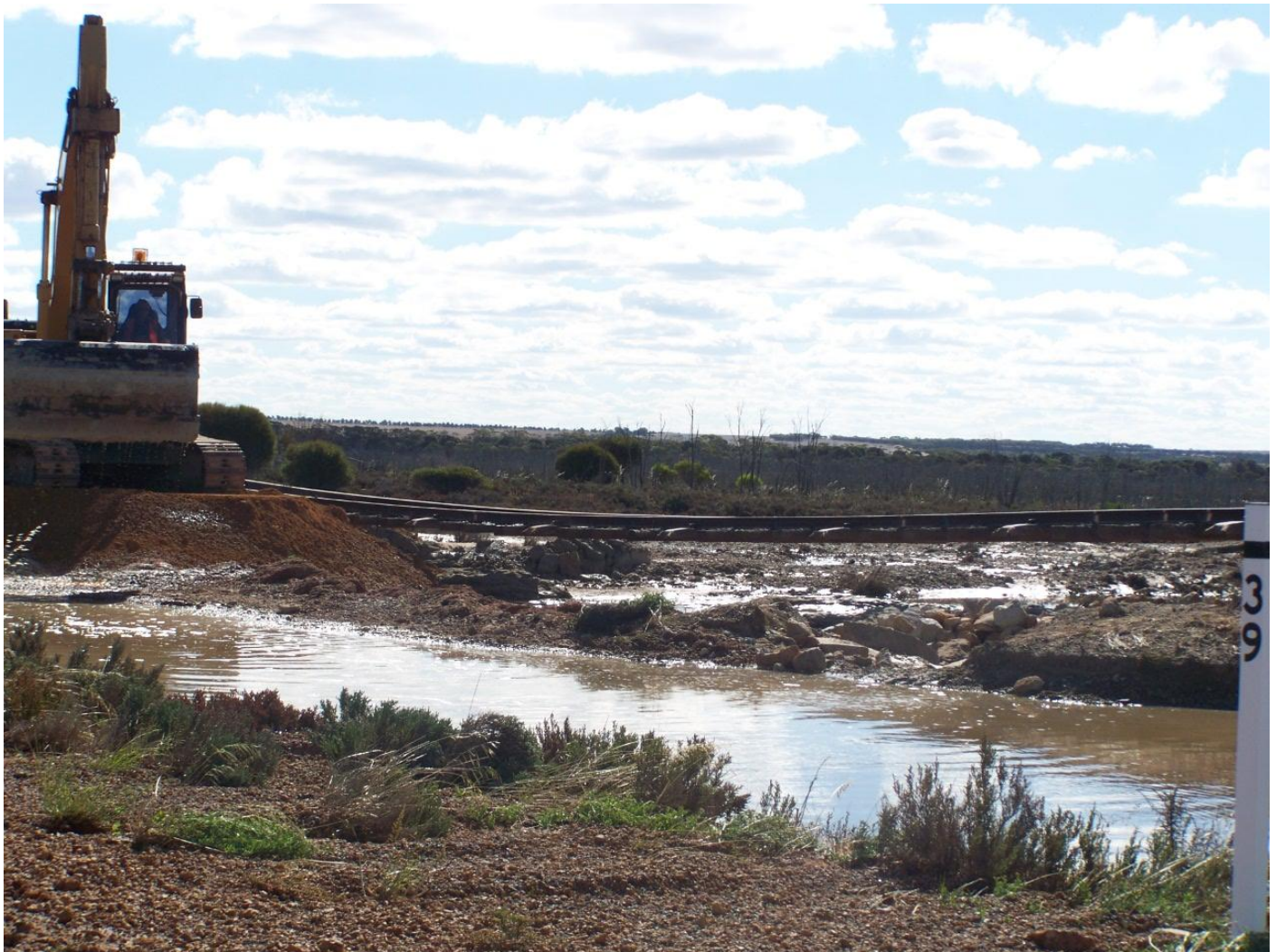
Commencing rebuilding the railway formation at Pingaring floodway December 10th. Photo Daryle Phillips
