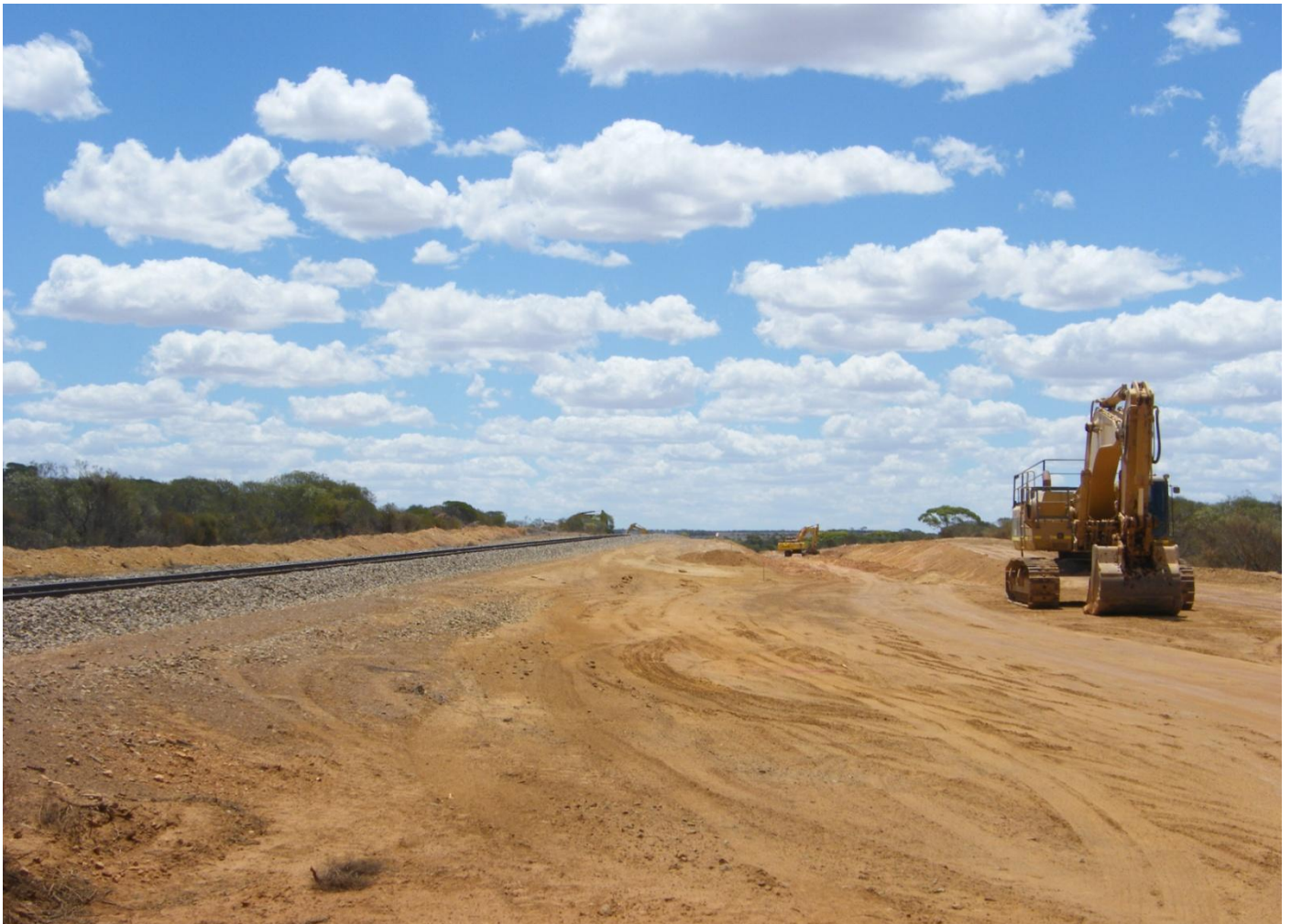
Earthworks underway on Perenjori line north of Tardun to improve gradient 16/12. Both photos Jim Bisdee
