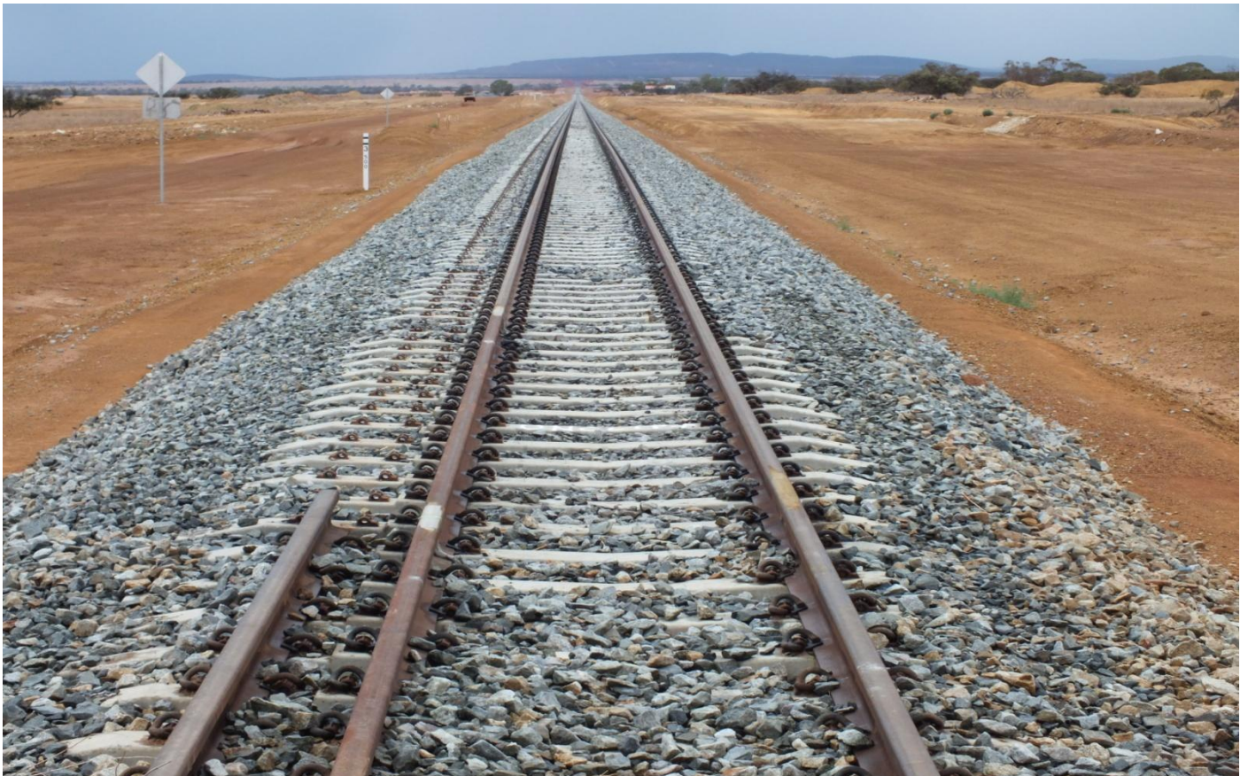
Regauged Karara line at Yalgoo Road crossing looking east March 24th.
