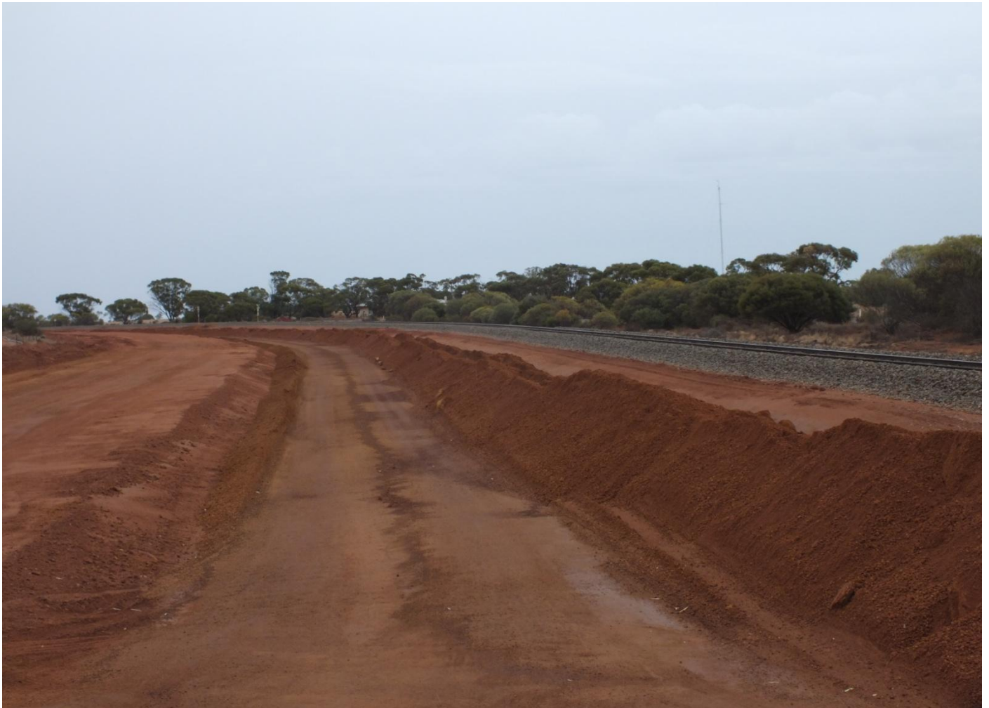
Earthworks to improve gradient in the Gutha area on Morawa line March 24th.
