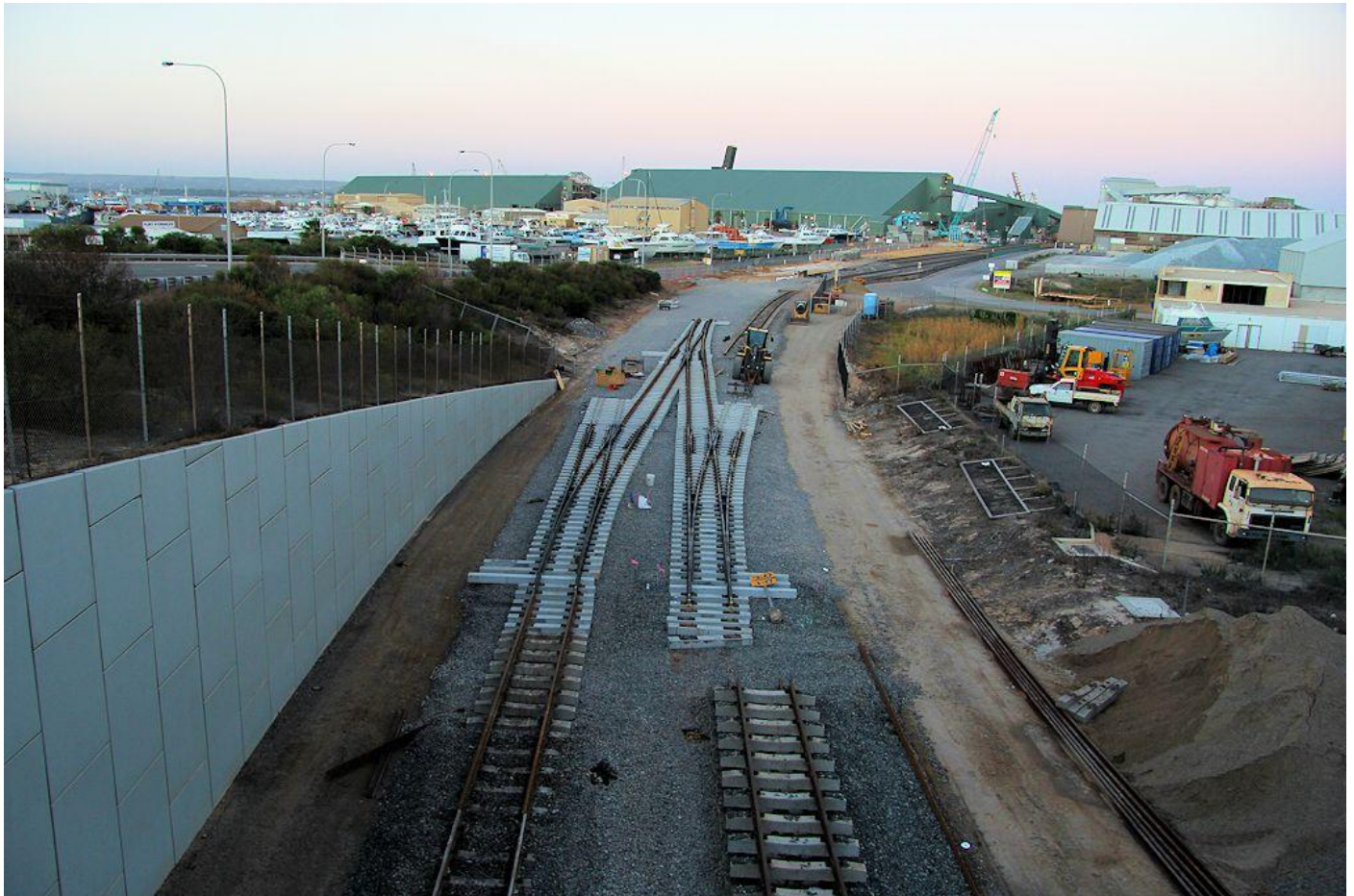
Track work underway at Port of Geraldton to increase from 2 to 3 tracks May 9th.
