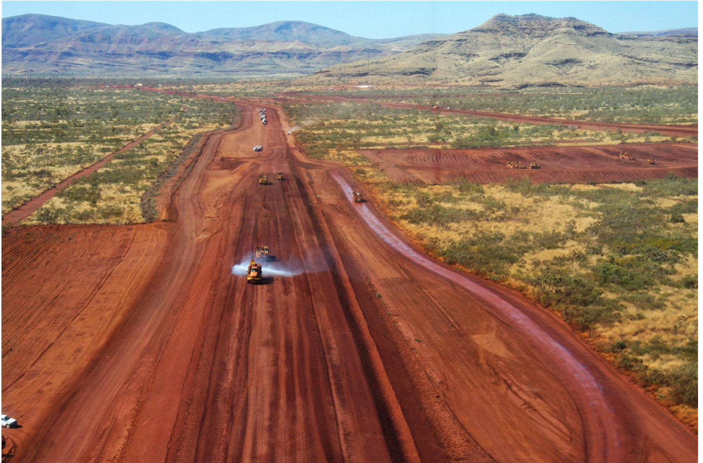
Construction of the new FMG Solomon mine railway line extension its formation under heavy earthworks looking east away from minesite along Hamersley Ranges May 21st. Both photos Don Copley
