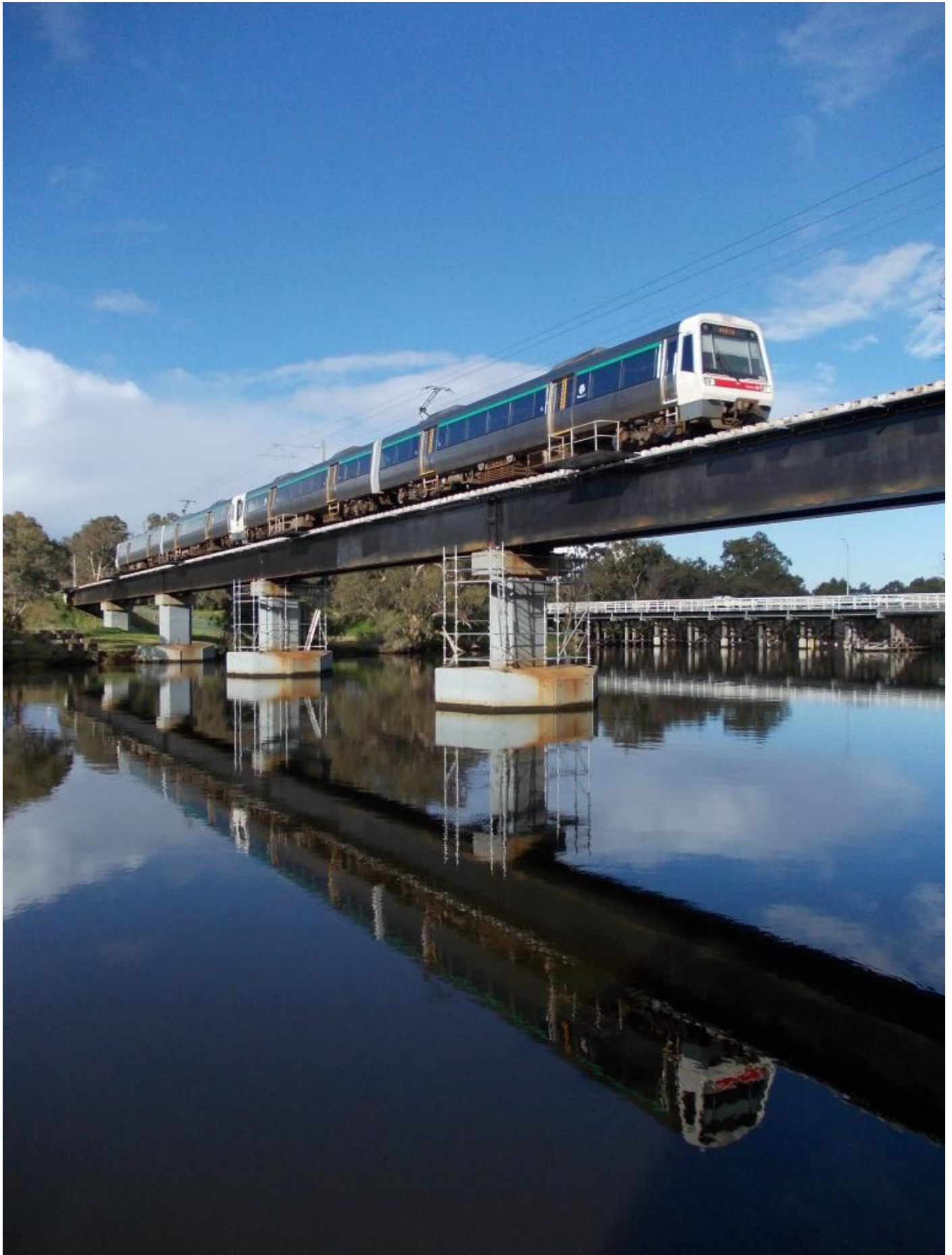
Four car EMU set crossing Swan River at Guildford August 1st on the original standard gauge steel and concrete bridge that was converted to dual gauge in 1974. Photo Mark Bennett. End page 12 of 12.
