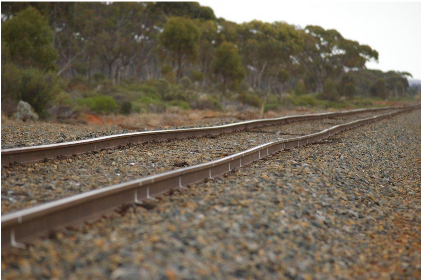
Leonora line just outside Kalgoorlie showing the track marked for sleeper replacement October 12th.
