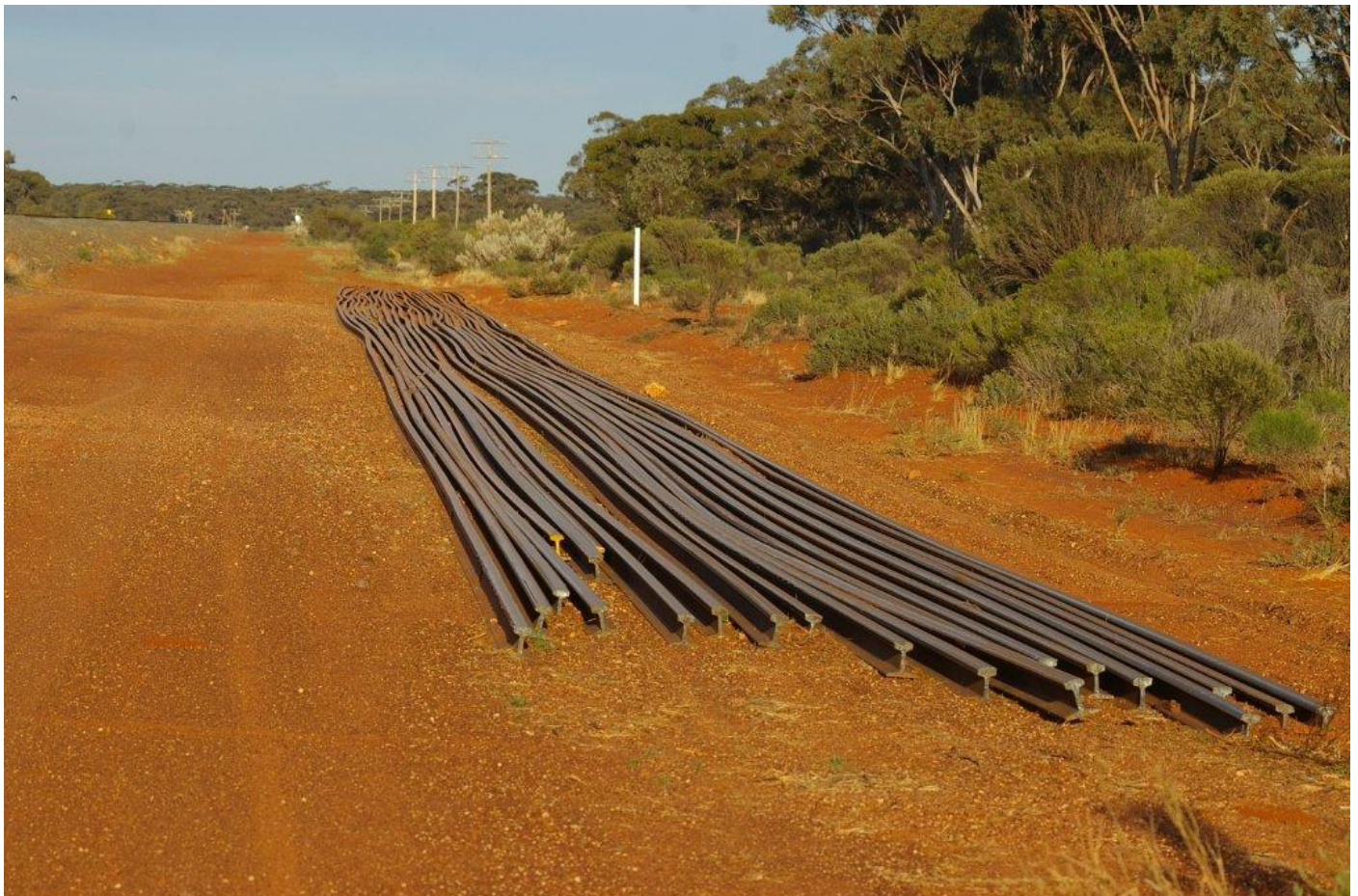
Strings of original 47kg rail recently replaced with 60kg plant as part of EGR upgrading laid out waiting recovery December 2nd.
