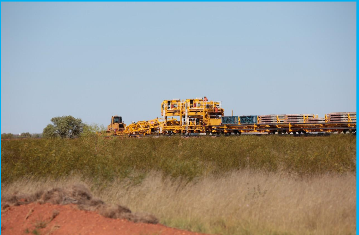
Tracklaying machine being used to lay Roy Hill railway on end of combined rail sleeper train 06/08.
