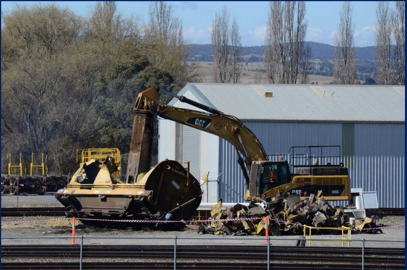
Aurizon AGWF [WAGR/Westrail XW] grain wagon being scrapped Goulburn NSW 15/8.
