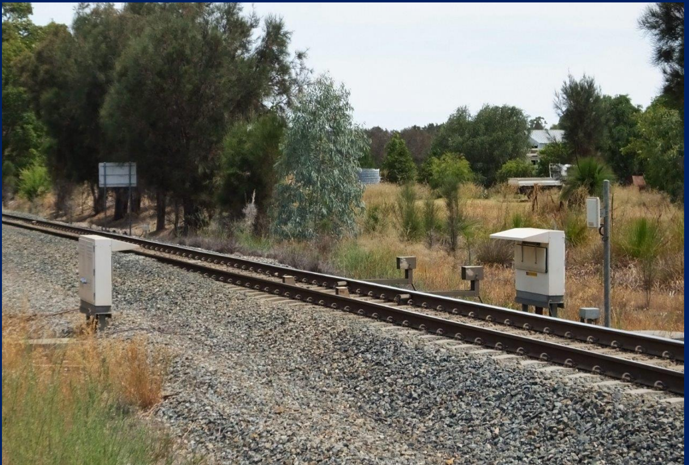
RailBam axle and bearing flaw detector from south side January 24th.
