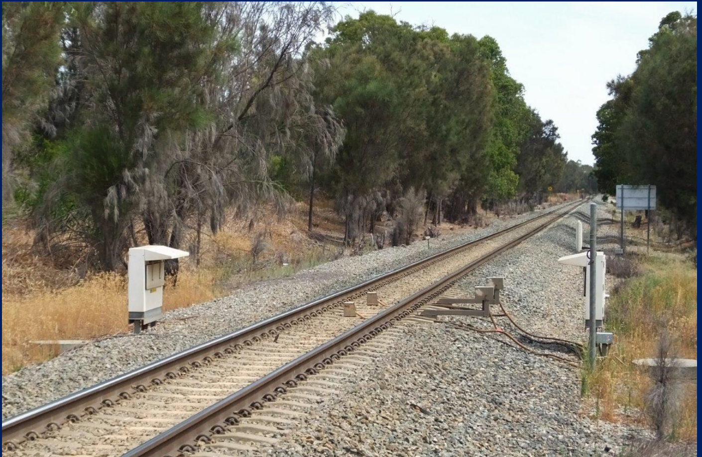
RailBam axle and bearing flaw detector south of Mundijong from the north side on 24th January.
