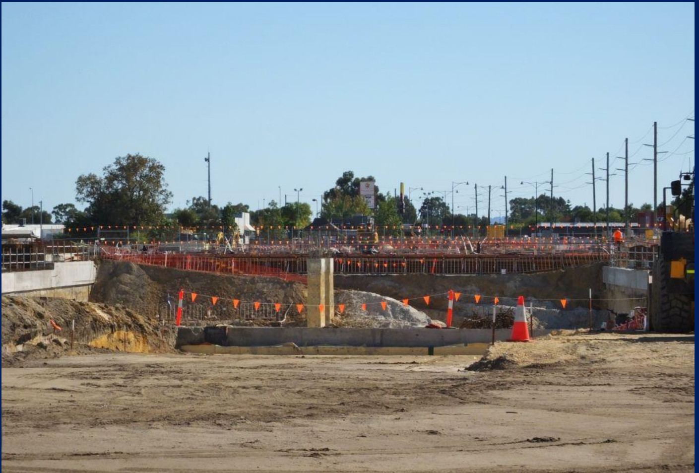
Grade separation works under way at Lloyd Street Midland with new up main bridge 6/4. Photo Jim Bisdee
