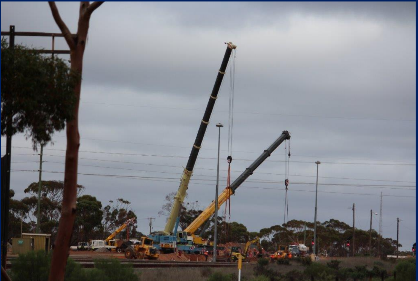
Two high capacity, heavy duty cranes lifting new turnouts into position west end West Kalgoorlie yard 19/4
