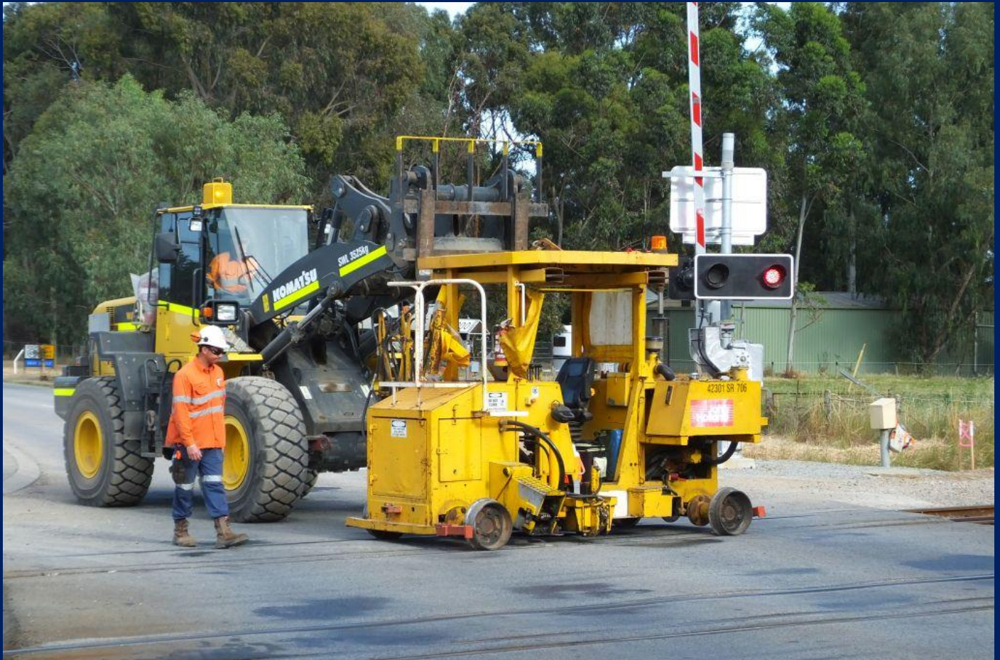
Sleeper replacer track machine being lowered onto track at Bushmead Road Woodbridge October 18th.
