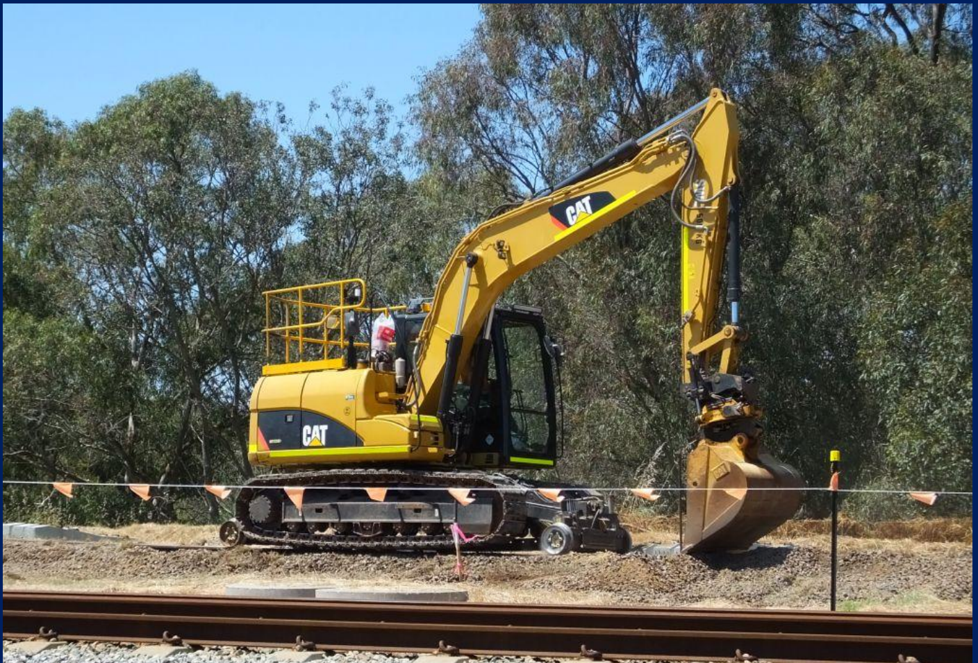
Excavator ballasting after sleeper replacement east leg Woodbridge triangle 20/10. Both photos Jim Bisdee
