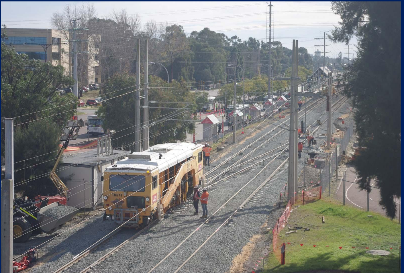
TM747 working on new turnouts at Cannington July 5th.
