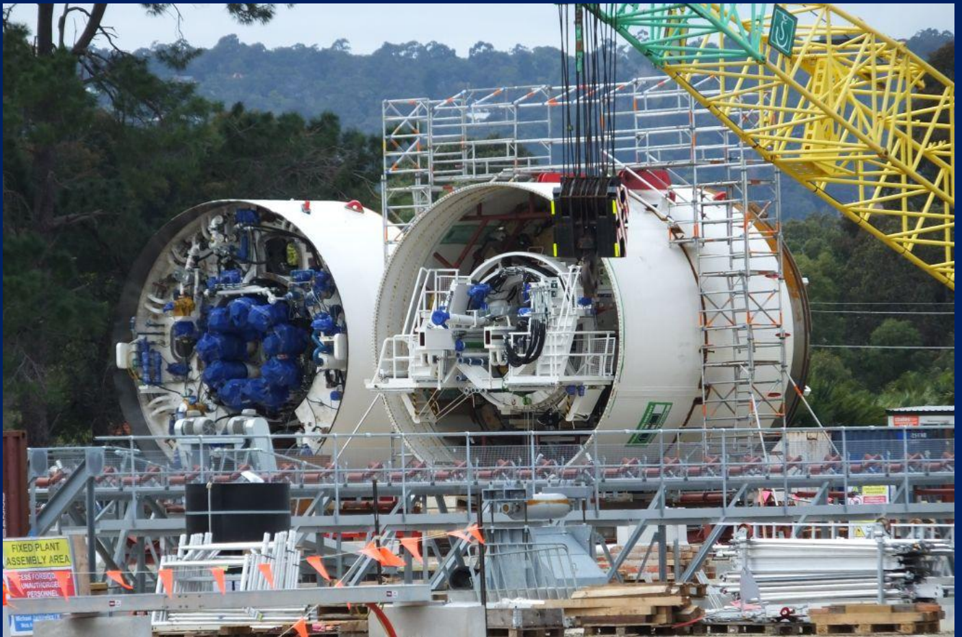
Second tunnel boring machine being assembled for use on Forrestfield line August 6th. Photo Jim Bisdee
