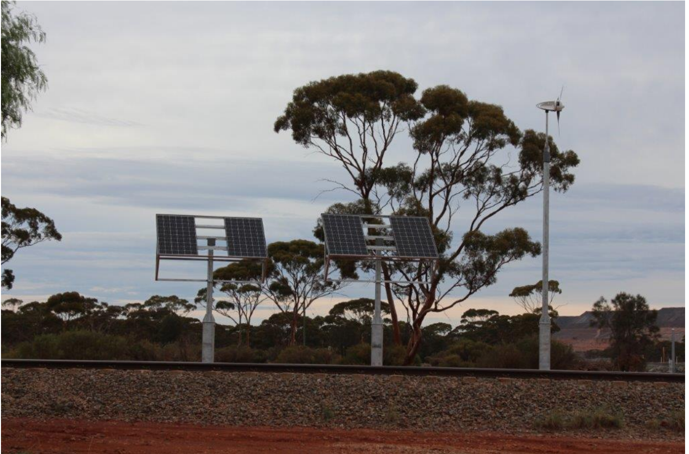
The new KCGM haul road crossing near Parkeston is now complete, with boom gates fitted. Solar panels and a wind turbine power this crossing. 21 st March. Both photos: Peter Donaghy
