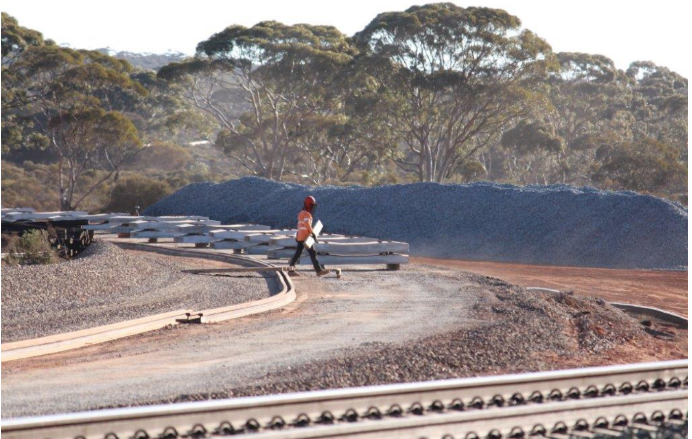
In late October, the east leg and south junction of Binduli triangle was cut, removed and rebuilt with concrete sleepers (previously all wooden) and new rails. 29 th October. Both photos: Peter Donaghy
